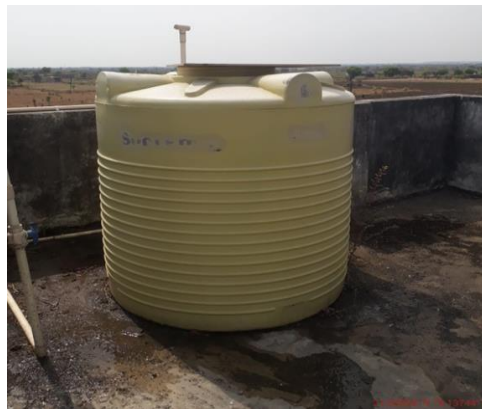
Overhead Storage tank
