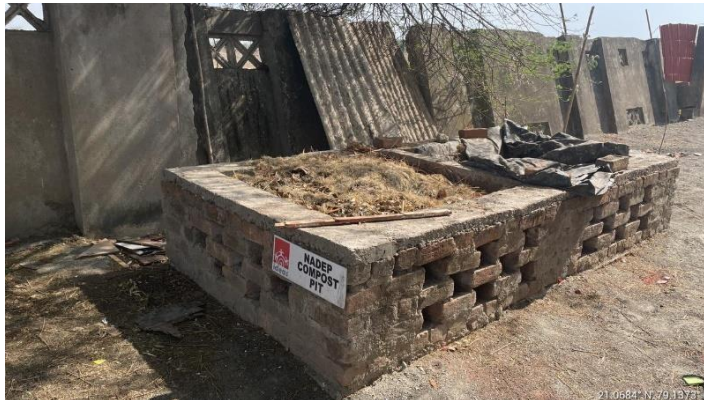
using the Nadep method in a two chamber pit
