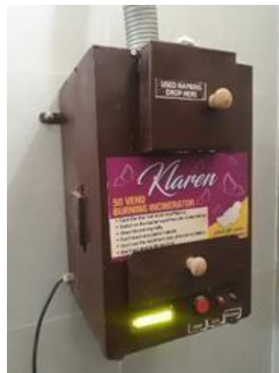
An Incinerator At Girl's Toilet
