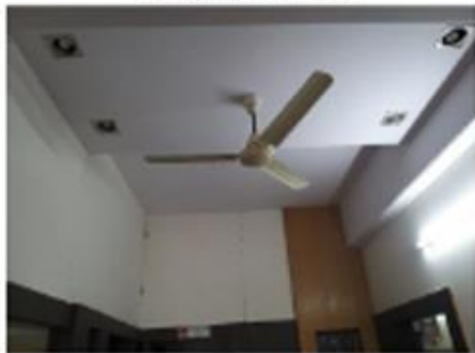
LED lights in Principal's Office
