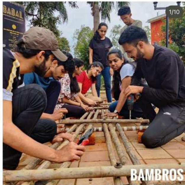
6.1 Students building a bamboo structure
