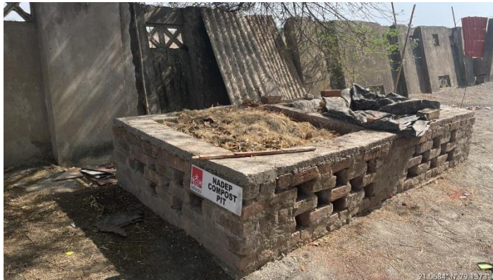
Dry leaves are composted using the Nadep method in a two chamber pit
