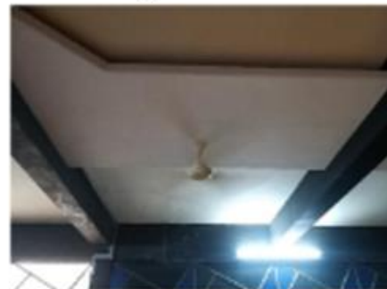
LED lights in Computer room
