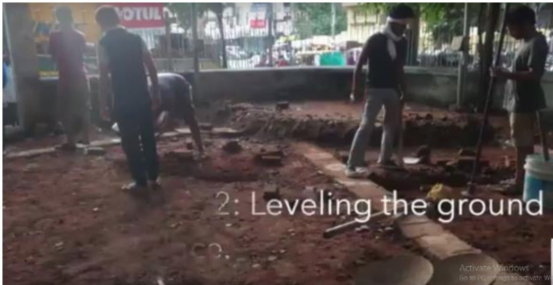
Phase II. Preparing ground for execution
