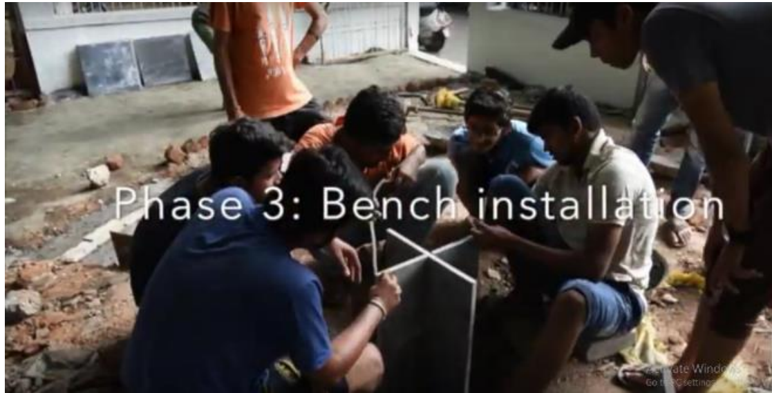
Phase III. Execution is progress
