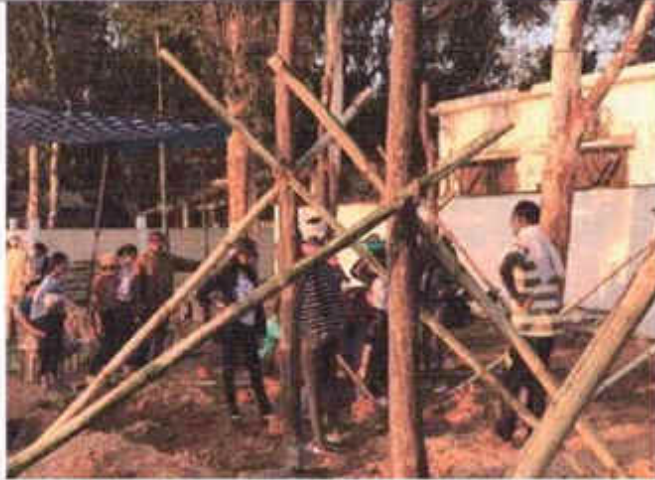
Building Construction Workshop at Khandgaon, Bastar 2018-19
