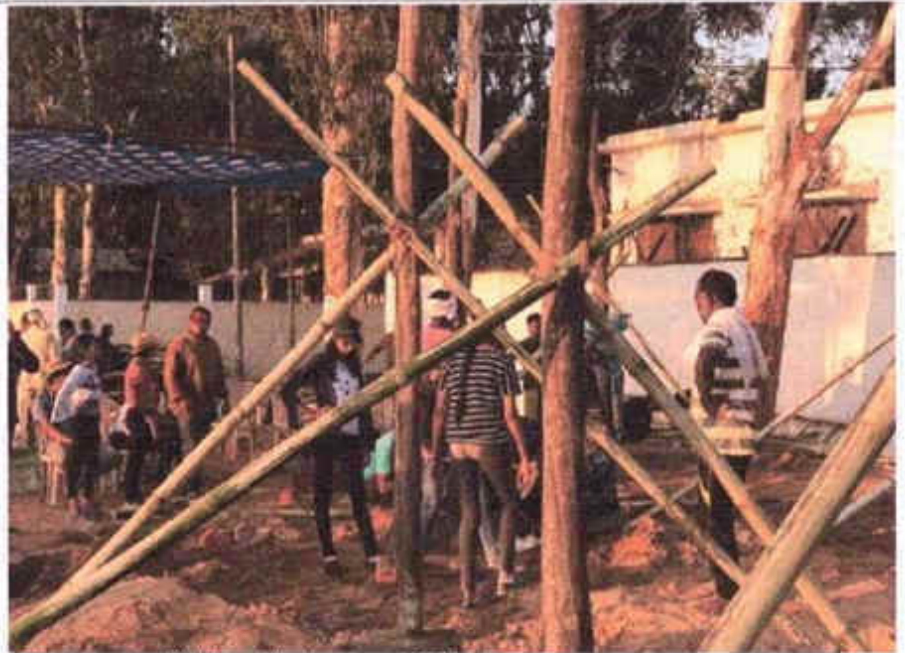
Building Construction Workshop at Khandgaon, Bastar 2018-19
