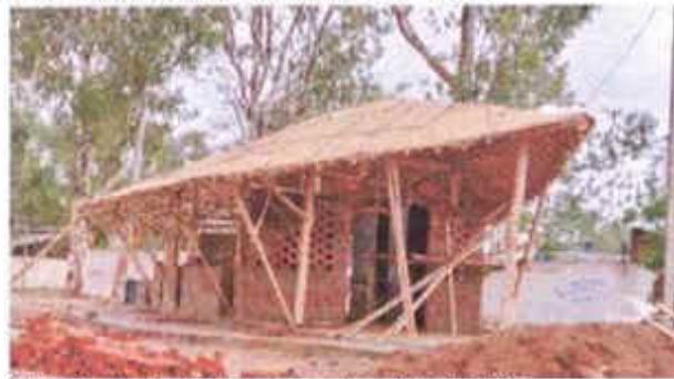
Building Construction Workshop at Khandgaon, Bastar 2018-19
