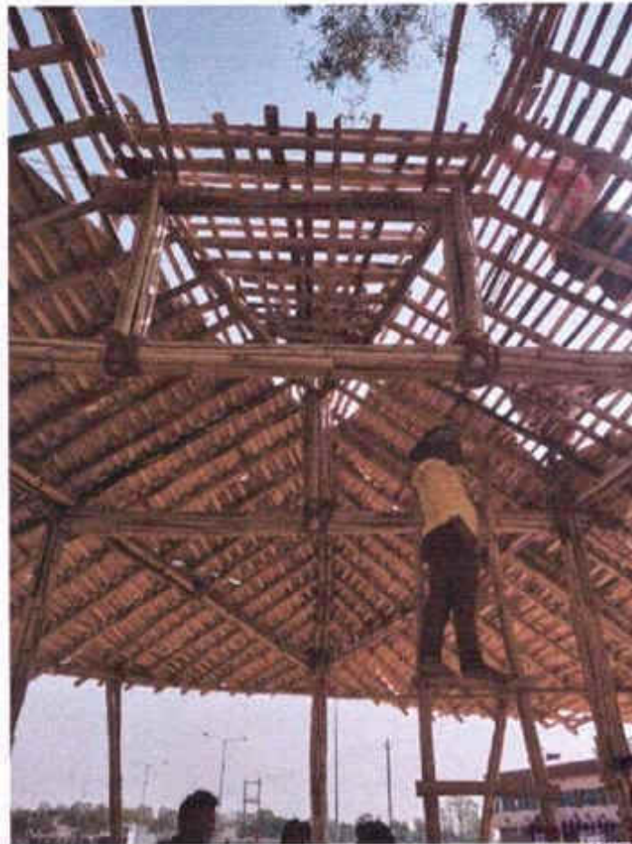
Building Construction Workshop at Khandgaon, Bastar 2018-19
