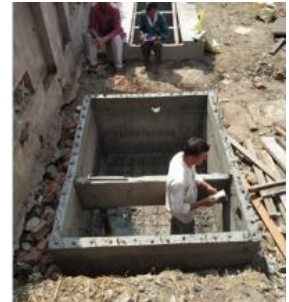
Figure 3 Septic Tank
