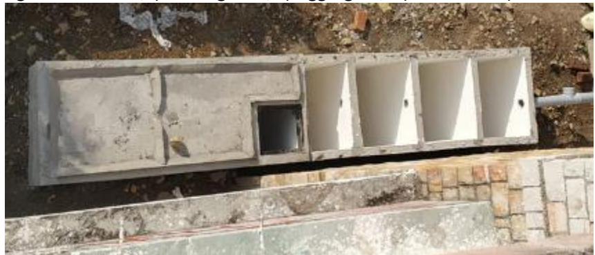
Figure 4 Four chambered anaerobic treatment tank
