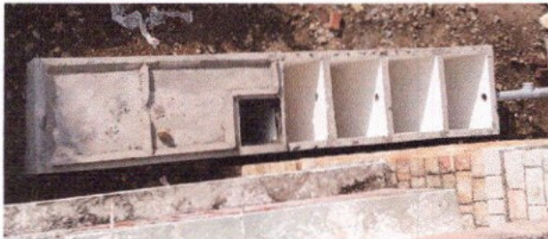
Four chambered anaerobic treatment tank
